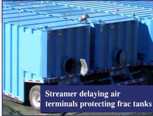
Streamer delaying air terminals protecting frac tanks
